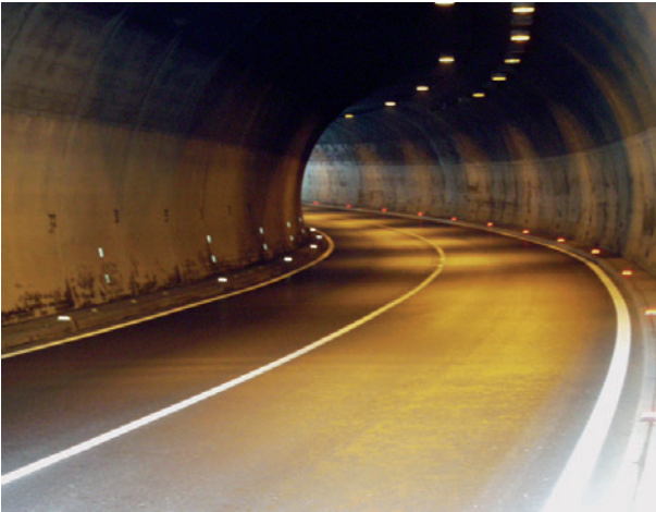
Kerb markings in tunnels
