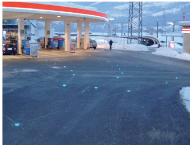
Lane marking for access roads and loading ramps
